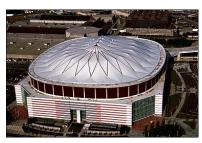
strength in architecture and building was based on rigidity and mass. That is, if an object fell on the corner of a wall built with bricks, the corner would absorb all the force and would crumble. If an object fell on the corner of a tensegrity wall, the whole wall would absorb the force and the wall would flex. Just as significant is the lack of a heavy support structure or anchoring mechanism
